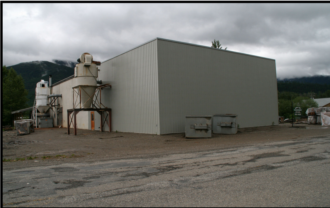
Top Front view with office/showroom Bottom Rear view with two dust collectors, 20 HP each, approx 13,000 CFM total
